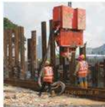
Installation of sheetpiles using vibro machine
