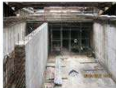
Tunnel walls casting completed 隧道牆建造完畢
