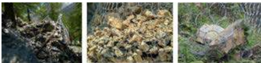
Fig. 1 Barrier capture of single rockfall and rock debris.
