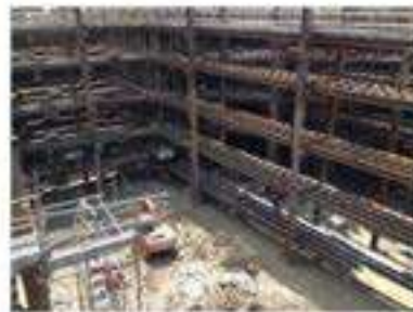
Excavation and installation of struts until formation level 挖土並安裝支柱達至地基面
