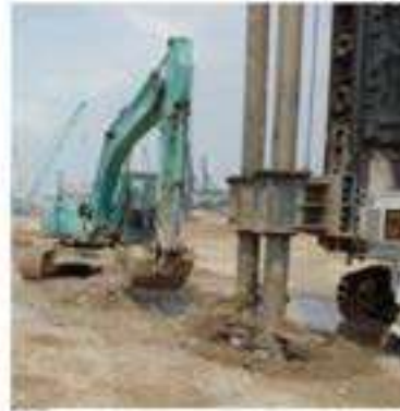
Soil Improvement works (injection of cement grout into the soil layer) 土質改良 (往土裏注入水泥漿)
