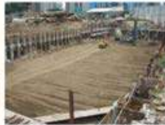
Backfilled to original ground level 回填砂土至地面
