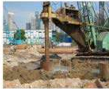
Installation of Foundation Bored Piles 安裝轉孔基樁
