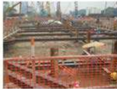
Stage by Stage Removal of Struts 階段性去除支柱
