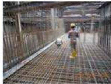
Arranging the reinforcement for the base slab 為底板的排列鋼筋
