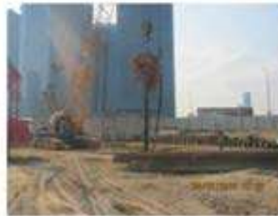
Removal of all Temporary Retaining Sheetpiles and Soldier Piles 去除臨時擋土板樁與支撐樁
